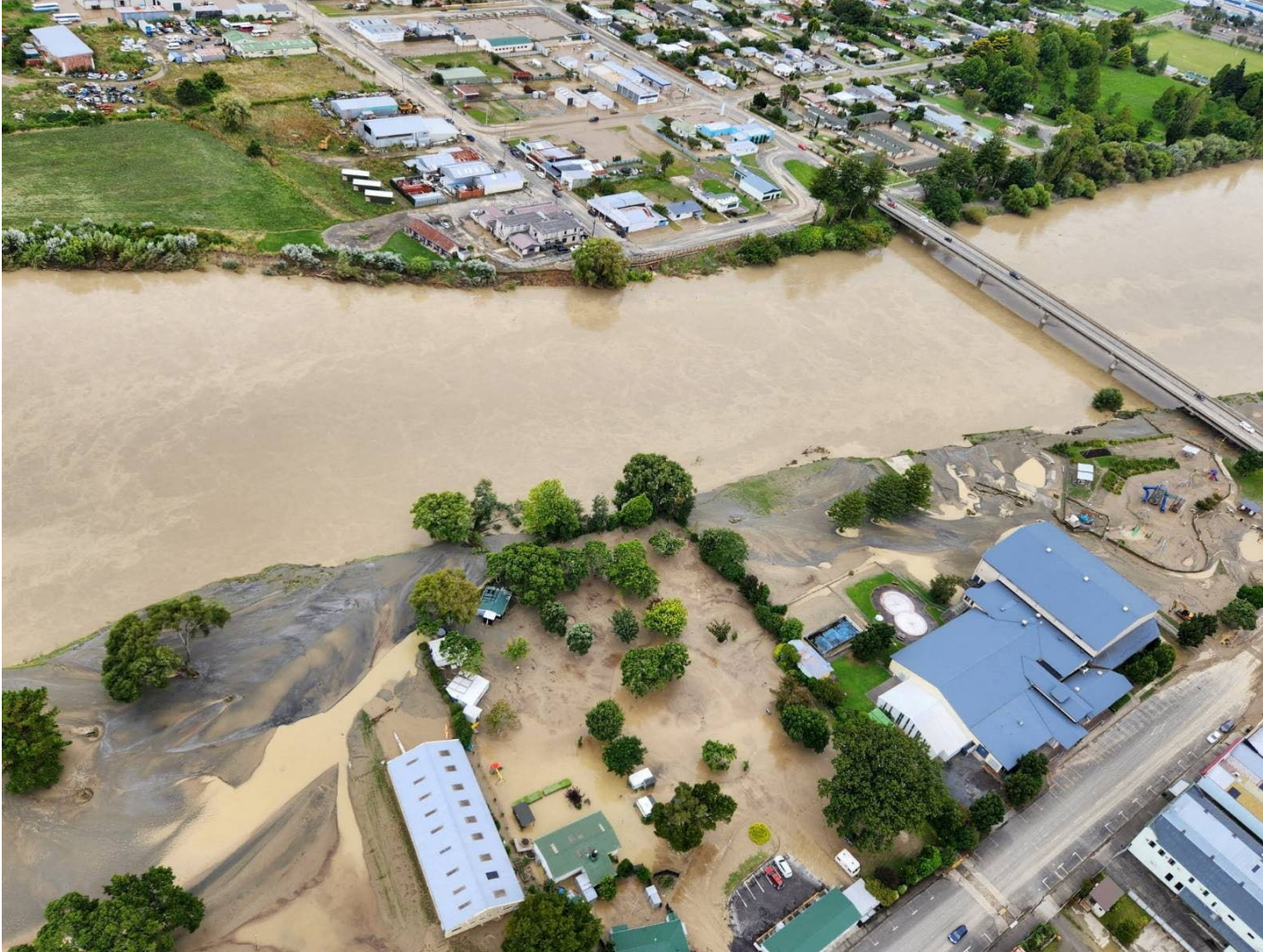
Image source: Reuters - A view of flood damage in the aftermath of cyclone Gabrielle in Hawke's Bay, New Zealand https://www.reuters.com/world/asia-pacific/new-zealand-police-still-looking-8-people-missing-after-cyclone-gabrielle-2023-02-25/
