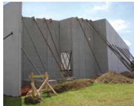
Photo: New data centre under construction.
