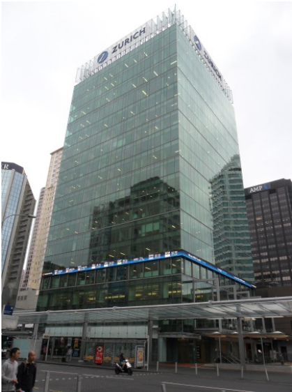
Figure 2: Existing commercial building in downtown Auckland with a floor plan 30m by 30m
