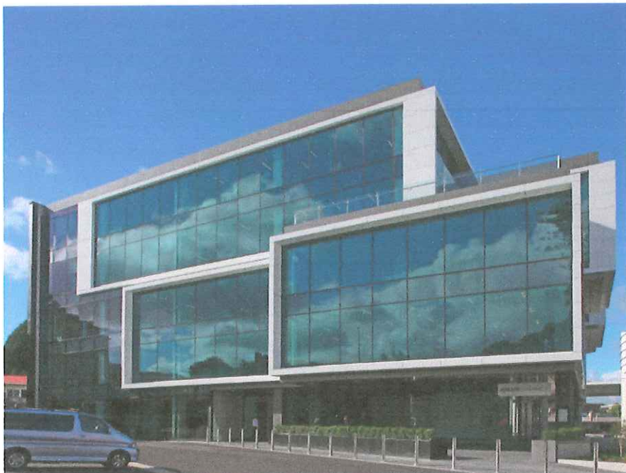
Figure 2: Watercare main offices, 73 Remuera Road, New Market
