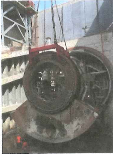
Figure 6: Observing Waterview Connection TBM Removal
