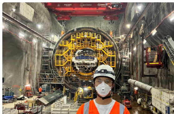
Eastern Busway Alliance Graduate on site at the tunnel boring machine.
