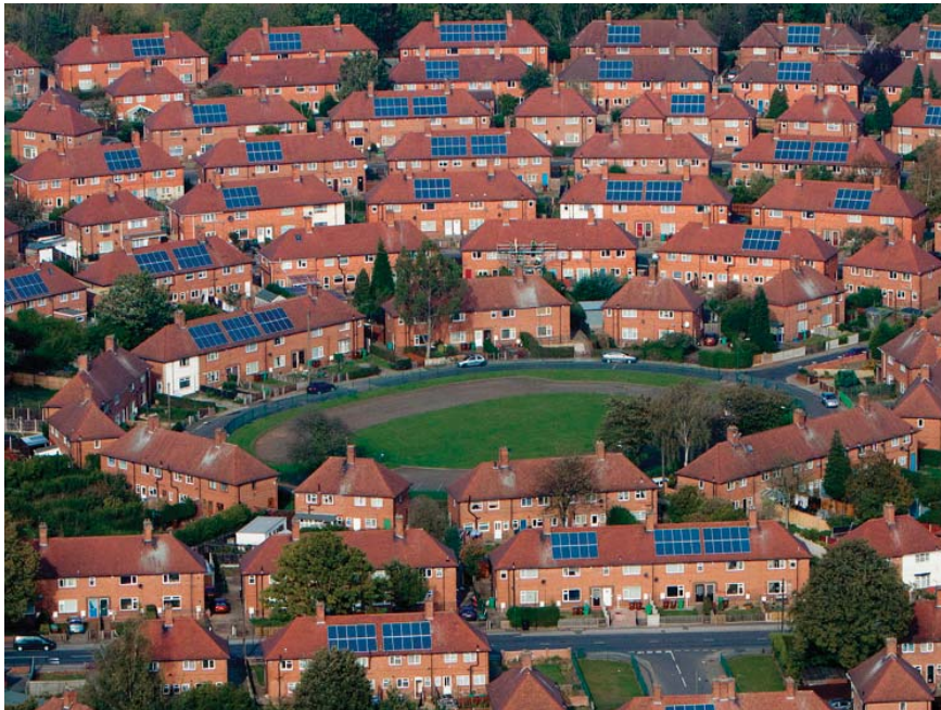
PV installations on social housing in the UK.
