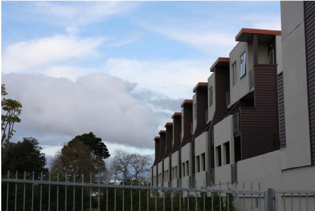
Figure 3.15: The Atrium on Main: View of development fronting the rail reserve area to the north, which in the absence of any development provides good outlook for these apartments (Source: Lee Beattie).
