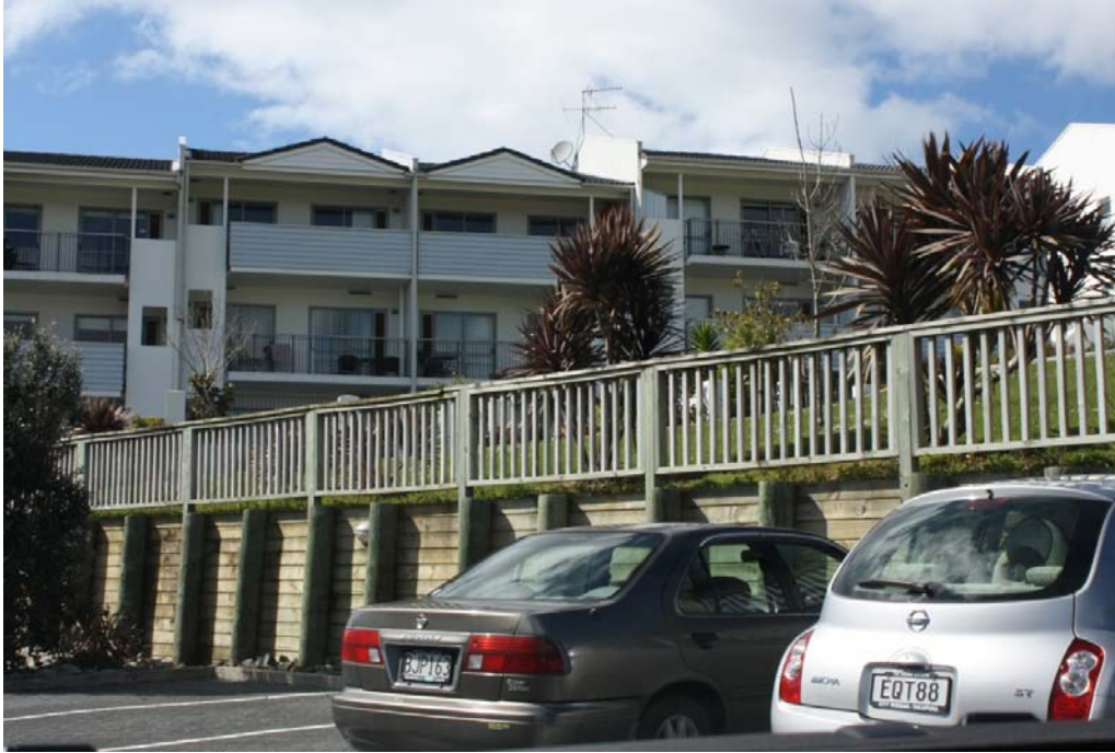
Figure 3.8: Masons Road, Albany: View of the development from McClymonts Road, looking into one of the ground-level car parking areas, with the communal open space beyond at a higher level. The considerable slope across this site is also evident (Source: Lee Beattie).
