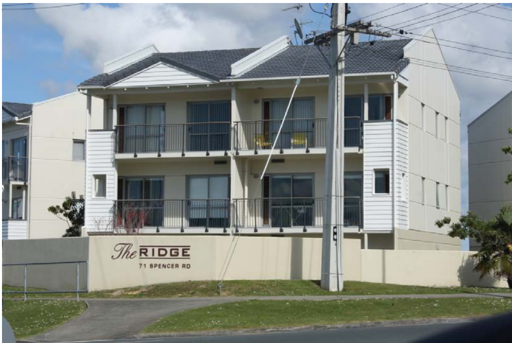
Figure 3.4: Spencer Road, Albany: Photograph taken from the corner of Spencer and McClymonts Roads and shows the typical dwelling construction used at The Ridge, with two residential units on each floor. It also shows the private open space allocated for ground floor units (set behind the perimeter wall) to the other units, with the first and second floor balconies above (Source: Lee Beattie).
