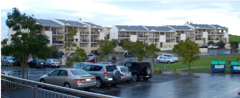
Figure 3.3: Spencer Road, Albany: Shows the extent of surface car parking and poorly positioned waste disposal facilities. The photograph was taken inside the development, looking towards the southwest corner of the site (Source: Lee Beattie).
