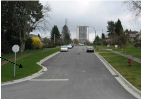
Figure 16 Bulged section along street
