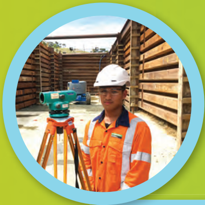
Alex | Army Bay wastewater pipeline, Whangaparaoa
