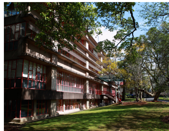
The main section of the Thomas Building, built in 1968
